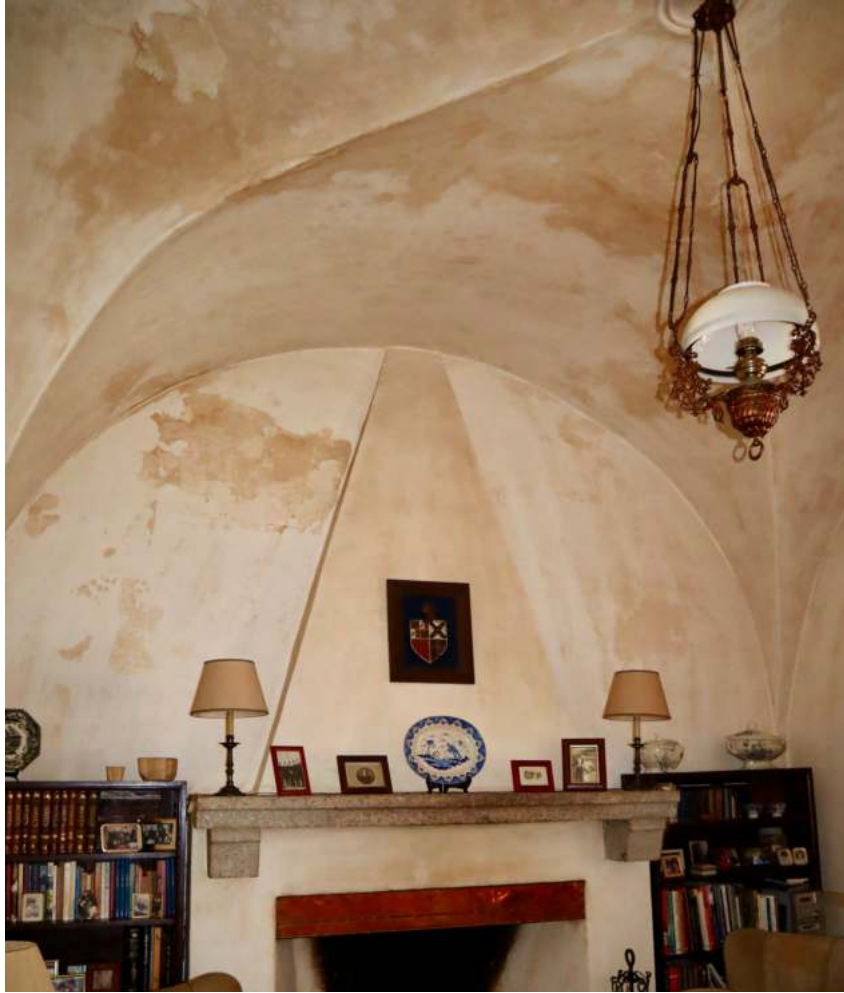
Fig. 14 Groin vaults in first-floor domestic spaces in Alentejo. Living room in Casa Rocha, Serpa. Source: authors, 2022.
