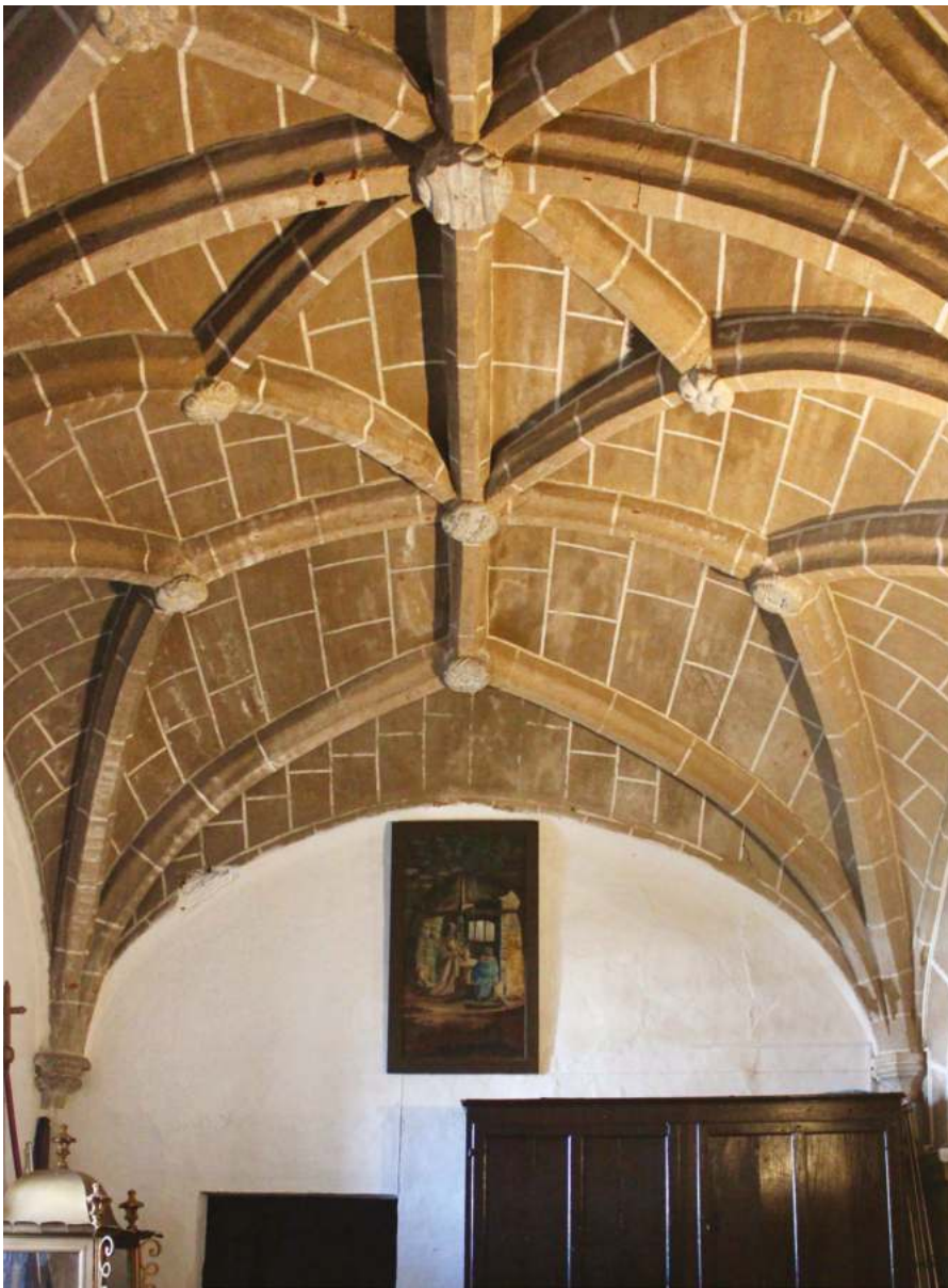
Fig. 24 Imitation of stonework. Sacristy of Convento do Carmo, Moura. Source: authors, 2023.
