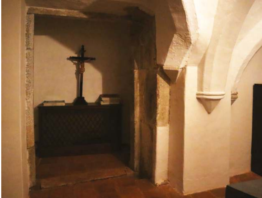
Fig. 25 Detail of irregular ribbed vault in Palácio Ficalho, Serpa. Source: authors, 2022.
