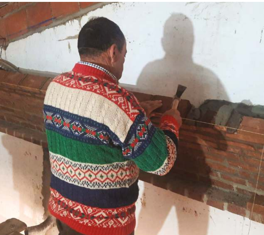
Fig. 2 A master builder at work during the construction of a vault in Baleizão. Source: Mafalda Batista Pacheco, 2023.
