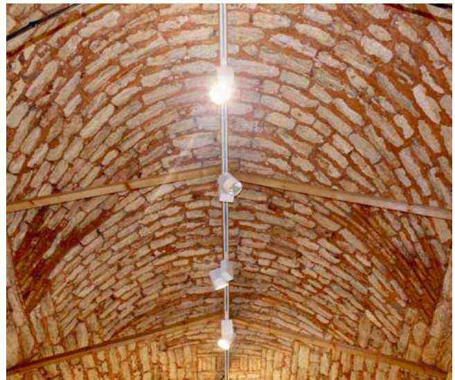
Fig. 7 Vault built with segments of pedra caliça in the same fashion as brick vaults. Shop in 3-5 Rua 5 de Outubro, Loulé. Source: authors, 2023.
