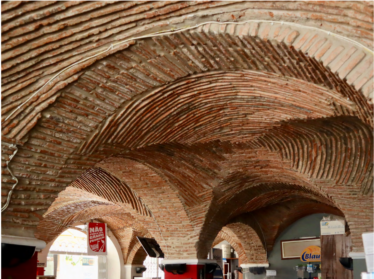
Fig. 5 Vault with bricks assembled perpendicularly to the intrados. Shop in Rua Cons. Augusto de Castro 11, Moura. Source: authors, 2023.
