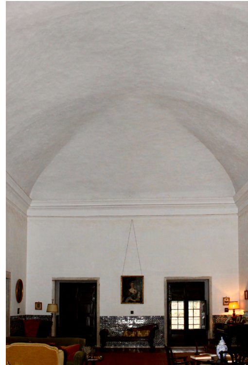
Fig. 16 Multi-span groin vaults in religious architecture. Cloister of Convento de Santo António, Loulé. Source: authors, 2023.
