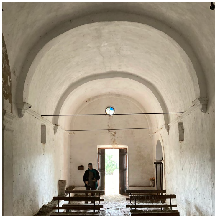
Fig. 9 Barrel vaults in ground-floor functional spaces. Cellar in Monte da Balsa, Portel. Source: authors, 2023.
