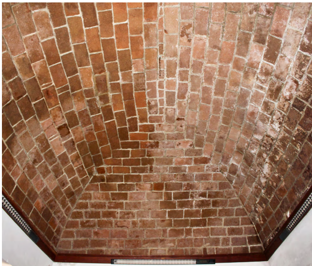
Fig. 6 Vault with bricks assembled horizontally/tangentially to the intrados (timbrel vault). House in Rua das Manhãs, Alvito. Source: authors, 2023.
