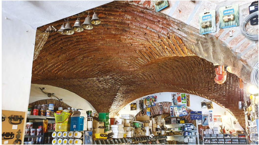
Fig. 5 Borba. Rua Marquês de Marialva 19. Four different ceiling structures in the same ground floor. The second and third compartments are covered by groin vaults; the front compartment shares an almost flat though timbrel vault, and timbrel vaults combined with metallic beams; and the side corridor displays a barrel vault. Source: author, 2024.
